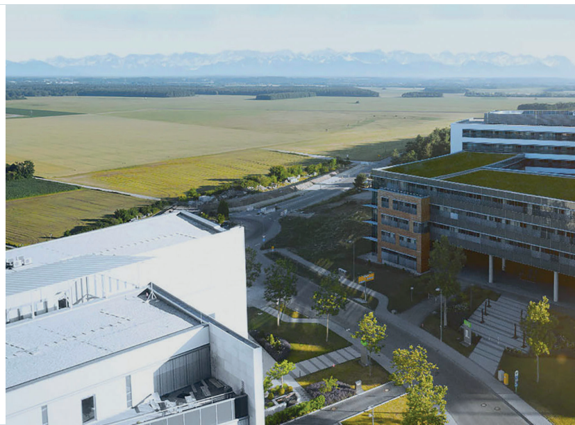
Condair location in Garching, Germany
